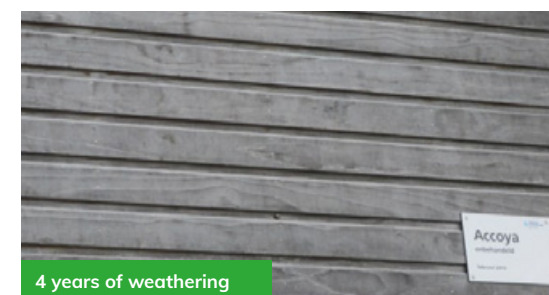
OFFICE CLADDING, VROOMSHOOP, THE NETHERLANDS
