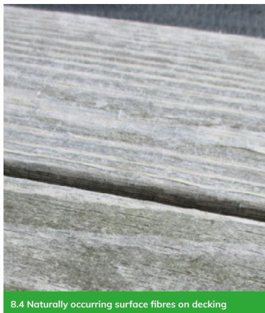
8.4 Fibres may get trapped in ribbed surface profiling
